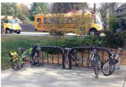
Rack does not allow use of a u-lock (Photo: Alta Planning + Design)
